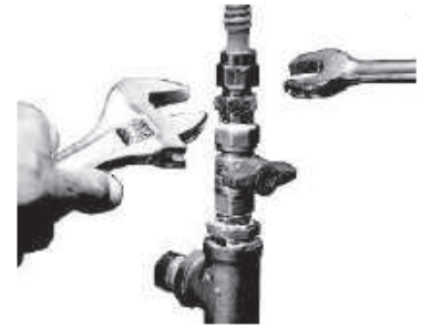
Always use two wrenches to tighten gas fittings
