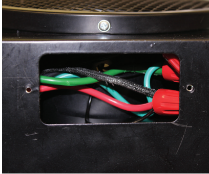
Figure 14: Wire connections carefully pushed into wiring compartment.
