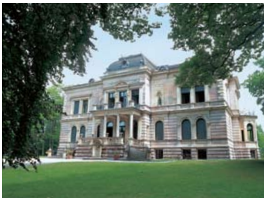
Administrative headquarters in the 1870s villa next to the Faber-Castell Castle
