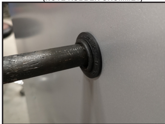
FIGURE 28 - FURNACE GAS PIPE CONNECTIONS (NOTE RUBBER GROMMET)
