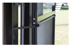
Custom anchors fit snugly into the screen door's inner channels while a pair of anchor screws hold it in place
