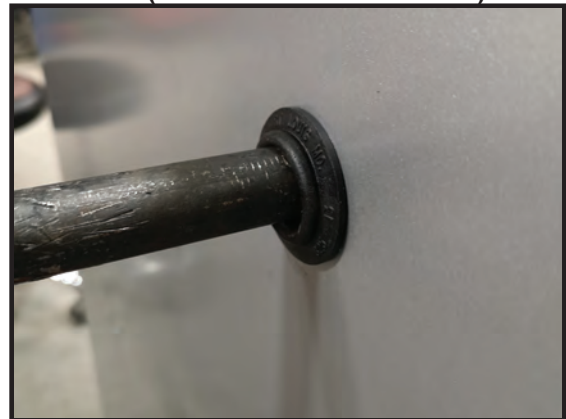
FIGURE 28 - FURNACE GAS PIPE CONNECTIONS (NOTE RUBBER GROMMET)
