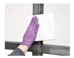
**STEP 1:** Align the materials — and make sure all surfaces are clean and dry. Use a 50:50 mix of isopropyl alcohol and water before applying tapes.
