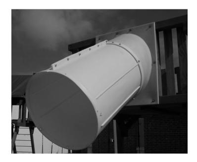
With a helper hold the Mounting Tube up against the playset tornado panel and align all sides with the panel. Attach using the 3" lag screws and washers.
