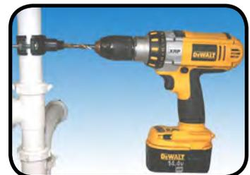
**Caution:** *It is very important to keep the drill centered to prevent damage of the drain saddle while drilling.*
