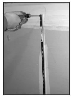
Rotate the wall bracket back into the vertical position and place screws in the last two holes and tighten. Don't forget to tighten the center screw that was left loose in Step 3.
