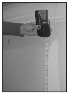
Using a tape measure, mark a spot on the wall 36 in. from the floor. This will be the location of the middle mounting hole and screw for the wall bracket.
