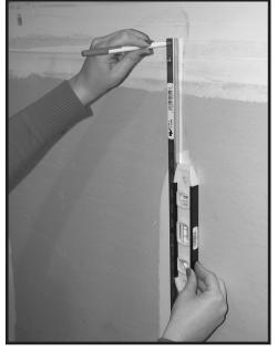
Using a level, align the wall bracket into the vertical position. Mark the location of the other two mounting screw points at both ends of the wall bracket.
