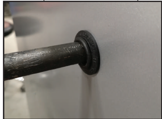
FIGURE 28 - FURNACE GAS PIPE CONNECTIONS (NOTE RUBBER GROMMET)
