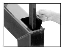
**Step 1**: Insert *Bird-Block* along one side of jack with the straight tab inside and the bent tab (with a pre-drilled hole) outside.
