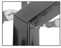
**Step 8:** Continue to hold pressure against *Bird-Block* and install a #10 – 16 x 3/4" screw through pole and bottom internal tab *Bird-Block*.
