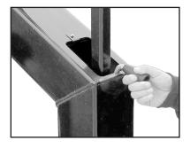
**Step 6:** Using a stick of wood or the handle of the jack, apply rearward pressure to bottom of internal tab of *Bird-Block* to keep it tight against back inside surface of pole.
