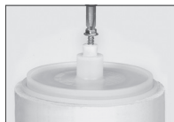
Ground-Rough Head Tests
