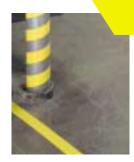
Yellow is used for marking physical hazards such as: low pipes, beams, handrails, pillars posts and fixtures that extend into work areas. Yellow is also used to warn against using equipment under repair. Solid yellow or yellow and black stripes can be used interchangeably.
