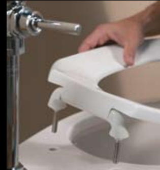
Assemble hinges.
