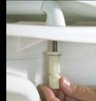
Center seat on bowl and finger-tighten STA-TITE® Fastening Nuts.
