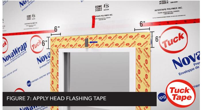
FIGURE 7: APPLY HEAD FLASHING TAPE
