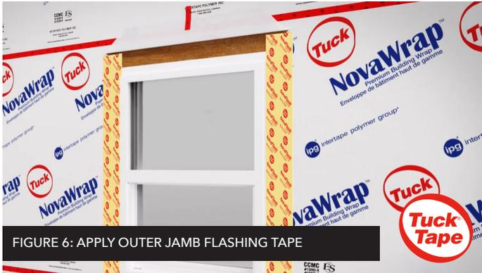
FIGURE 6: APPLY OUTER JAMB FLASHING TAPE
