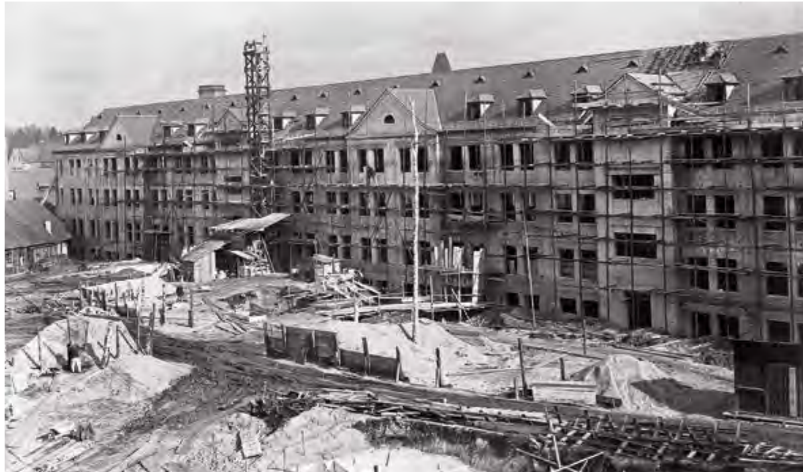
The manufacturing plant under construction, 10 March 1926
