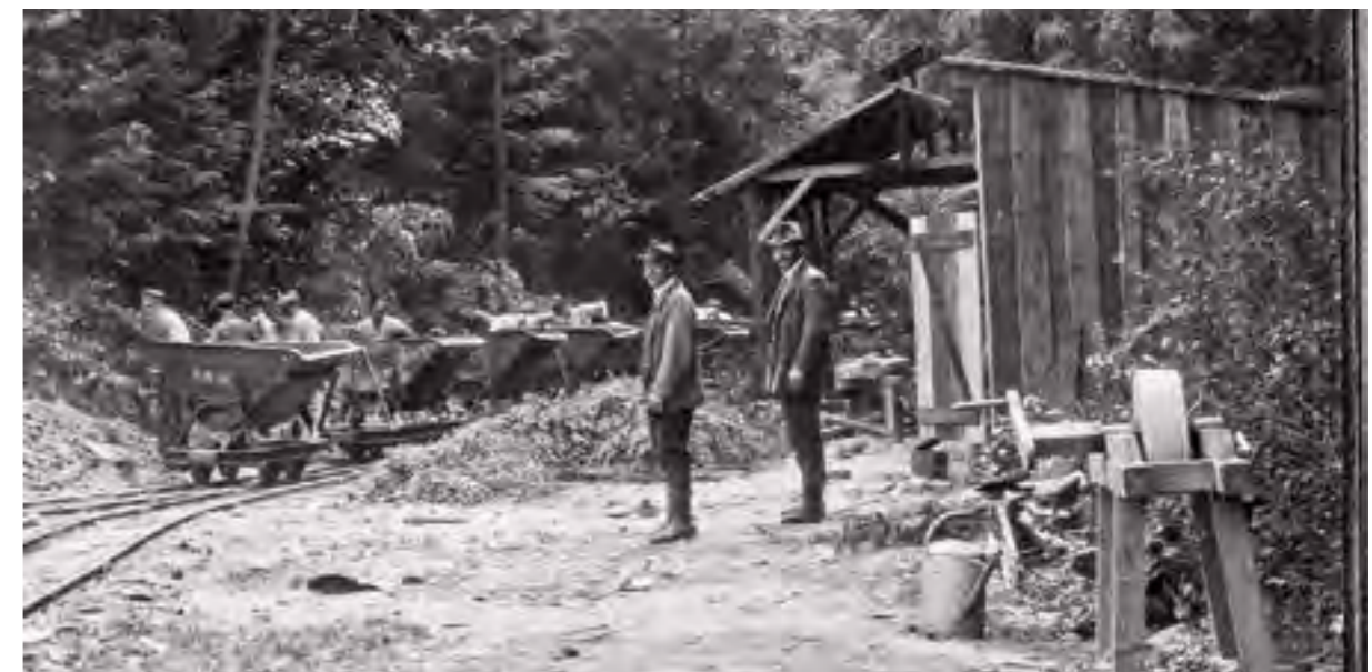
Excavating for the new factory building in Stein, 15 and 30 June 1925
