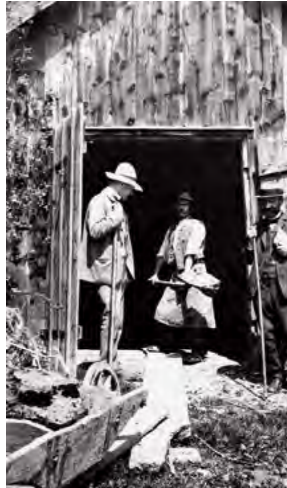
In pits and shafts at a depth of six to seven metres, the clay is arduously dug out and lifted to the surface with shovels on a step-like scaffolding and then pounded down into wooden barrels.
