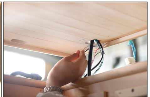
\*While placing the roof over the sauna, feed each of the heater cables on the side and back walls, and the wire harness and power plug in the back left corner, through the corresponding holes on the perimeter of the roof.
