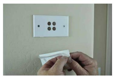
5. Starting at one corner, align the long edge of the rubber face to the indent on the S-Mount. Adjust as necessary. Once the alignment is perfect, then press the edge onto the S-Mount.
