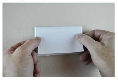
Remove the remaining backing from the rubber face. Carefully attach the remaining face rubber, lining it up with the edges as you work your way across. Be sure to press out air bubbles as you attach the rubber.
