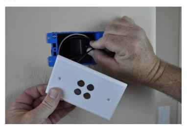
3. Using the supplied #2 Philips head screws, mount the plate. Make sure the S-Mount is tight to the wall. Do not overtighten and bend the S-mount, the face should remain flat.
