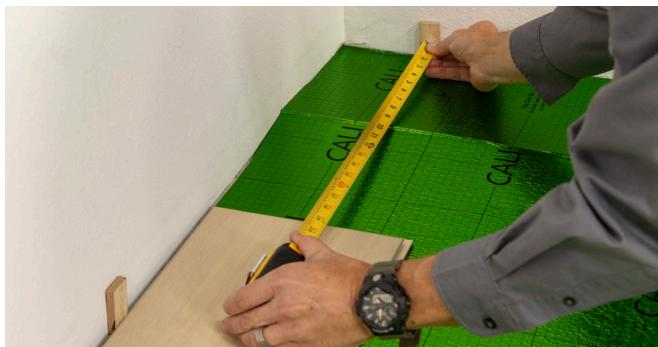
3. Cut the final board piece to length and install it in the same manner as the previous piece. Use the extra cut piece to start your next row if it is longer than 8".
