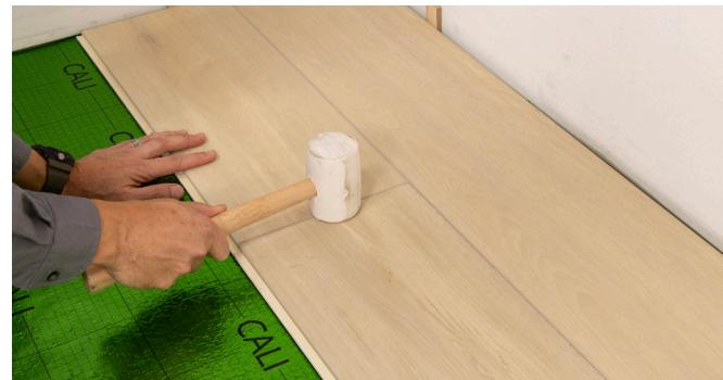
8. Make sure both planks lay flat afterwards and that all seams are tight. Use of a tapping block along the long side of the planks may help to ensure secure engagement. Continue installing the rest of the planks of this row.
