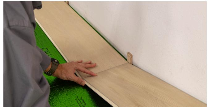
2. Install the second piece by aligning the butt end with the end of the first piece at a 45 degree angle. Gently push the second piece down until the tongue and groove lock together to secure the joint on the ends. The planks should lay flat. Continue in this manner until reaching the final board in the first row.
