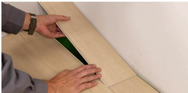
10. The last row may need to be cut lengthwise (ripped). Cut the last board to size. Use a pull bar to engage the length of the last plank.
