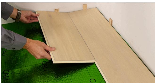
4. Confirm the first row is straight. Install the first board in the next row by angling it up slightly, pushing forward and interlocking the long side. The long side of the plank should fit snug with no gapping.
