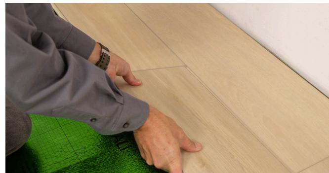
7. Slightly lift the second plank and push in slightly along the length of the butt seam until the long side is fully engaged. The adjacent plank will also lift. The butt end seam should stay engaged during this action.
