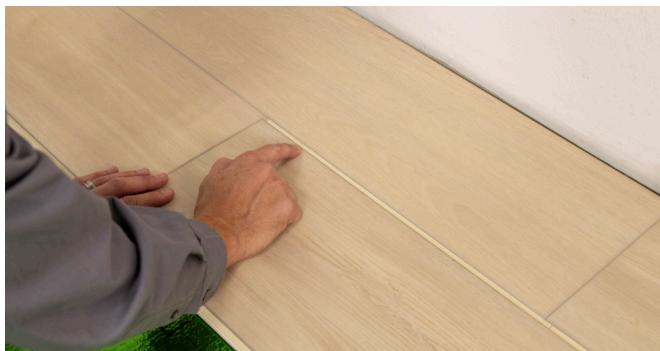
6. Insert the butt end of the second plank into the butt end of the first plank. Offset the planks by about 1/2."
