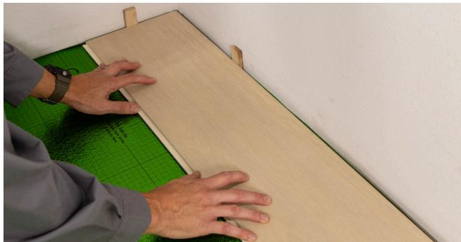
1. Starting from the left with the tongue-side facing the wall, carefully lay the first board in place, using spacers to leave an expansion gap between wall and edges of the plank.
