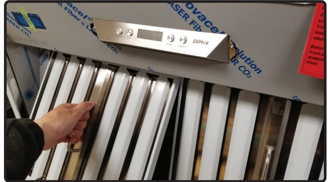
2. Remove baffle filters and duct covers from range hood.
