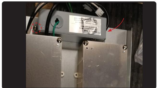
18. Secure the electrical box by (2) screws.
