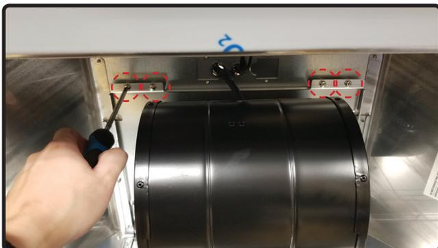
5. Remove (4) screws from the interior of the hood body attaching the single blower plate to the top of the hood body. Remove single blower and single blower plate.
