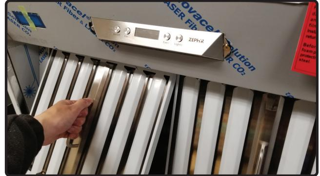
20. Install baffle filters and duct covers back onto the hood.
