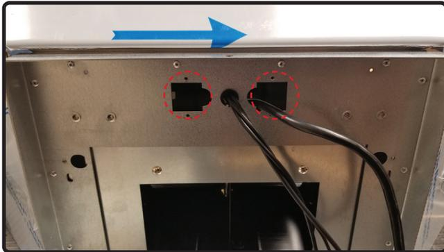
13. Secure the wires to hood body with the wiring hole covers by (2) screws each.
