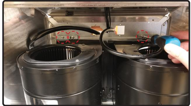
8. Position the dual blower bracket with the dual blowers into the hood body as shown. Make sure to tuck the dual blower plate into blower plate tabs. Secure the dual blower bracket by (4) screws.
