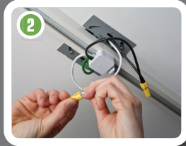
Connect track to mounting plate and wire.
