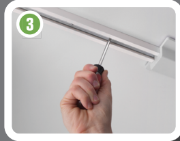
3 Attach track to ceiling.
