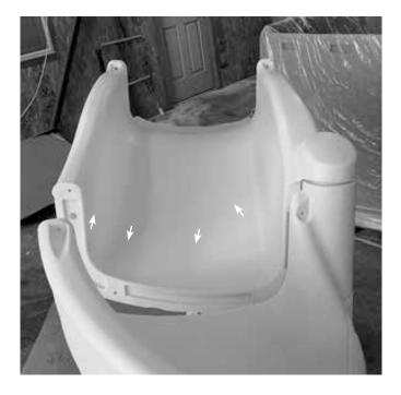
**4.** Attach entry section to last curved section using 3/8" x 3" stainless steel lags (DO NOT OVERTIGHTEN!).
