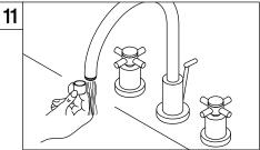
11. Remove the aerator, turn on the faucet, let water run for at least one minute, this will clear any debris left in the line, reinstall aerator.
