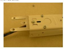
6. Reinstall channel cover assembly and lens.
