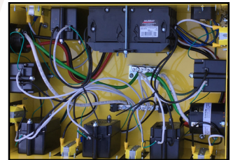
Image A is a Southwire Box. Everything is zip tied and tied down. Image B is competitor, some are zip tied but nothing is tied down. Messy appearance.
