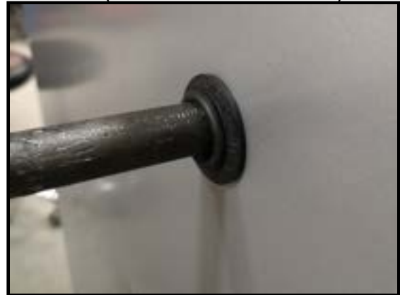
FIGURE 28 - FURNACE GAS PIPE CONNECTIONS (NOTE RUBBER GROMMET)
