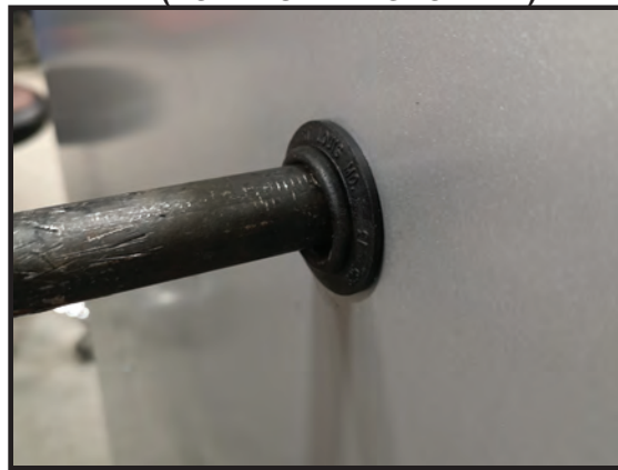
FIGURE 28 - FURNACE GAS PIPE CONNECTIONS (NOTE RUBBER GROMMET)
