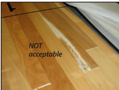
Play surface must be smooth and level with NO dips over 1/32" in depth and NO visible filler (see photo above).
