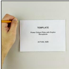
Using the template supplied (see page 5 of instruction sheet), trace the opening for both the top and bottom plate. See Figure 1 before tracing your opening. Remember, the plates are designed to be mounted centered between the studs. Using a drywall saw, cut a hole in the drywall the size of each template.
