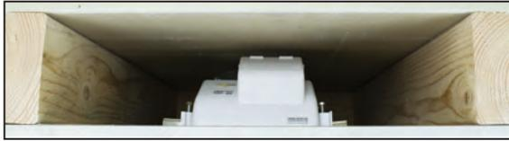
**Top view** - shows needed space between the drywall and the studs. The power output plate should be centered between the studs.
