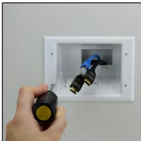
Using a Phillips screwdriver, tighten the screws with wings. These wings fasten tightly against the back of the wall. **Note:** Do not overtighten screws.
