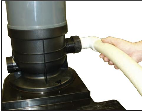
Figure 21 — Attaching flex pipe to filter
