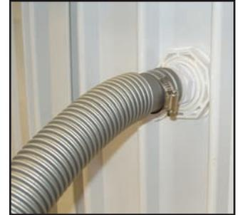
Figure 17 — Free end of hose attached to return
