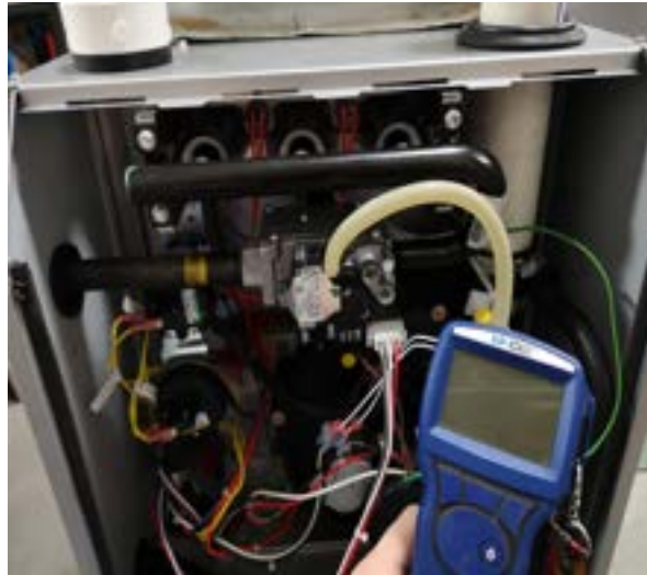
FIGURE 30 - MANOMETER MEASURING GAS MANIFOLD PRESSURE
