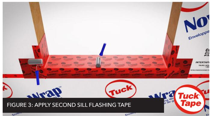
FIGURE 3: APPLY SECOND SILL FLASHING TAPE
