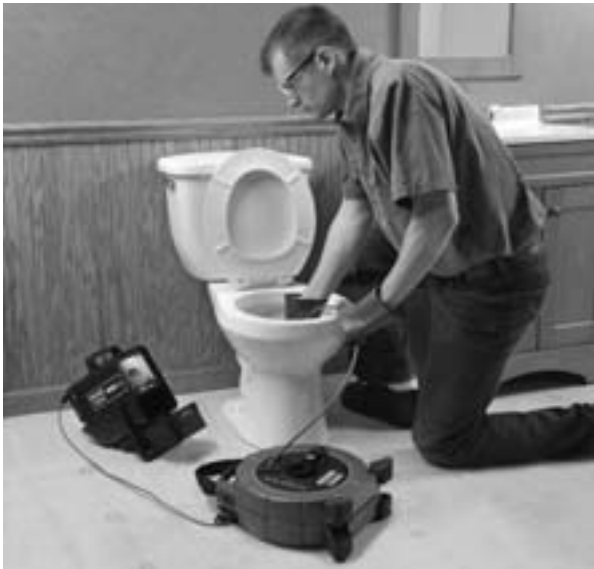
Figure 15 – Doing An Inspection
