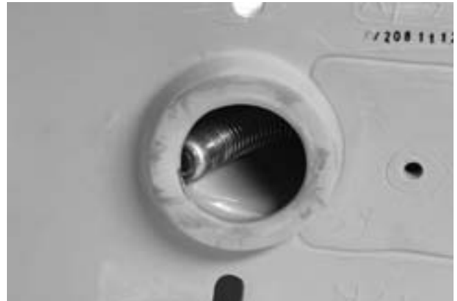
Figure 20 – Camera Head Blocked in Turn
