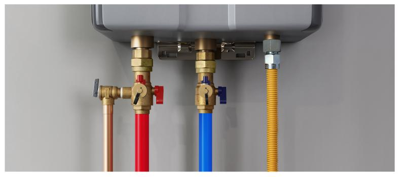
Jones Stephens' Tankless Water Heater Kits provide quick and simple installation. These convenient kits include high-quality forged brass valves and select models include a pressure relief valve, and gas connector – all in one box.
