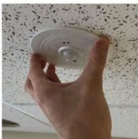
8. After the batteries have been installed for at least 3 minutes, initiate the Installation Test Mode: Momentarily press the Utility button. The green LED flashes once then the red LED flashes each time the sensor detects motion. (The test mode times out after 5 minutes).
