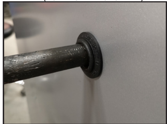
FIGURE 28 - FURNACE GAS PIPE CONNECTIONS (NOTE RUBBER GROMMET)
