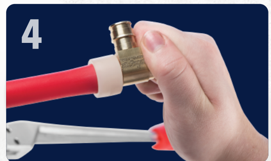
Insert the connector and let the PEX contract
