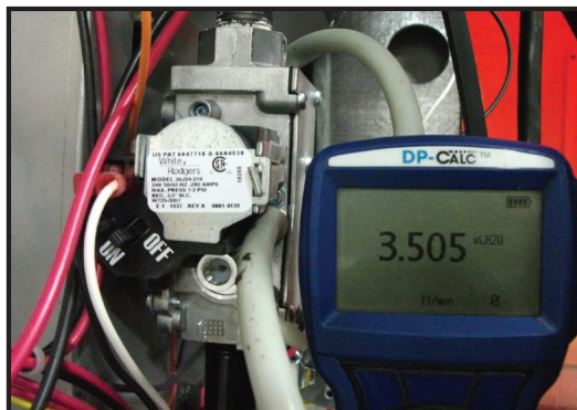
FIG. 30. - MANOMETER MEASURING GAS MANIFOLD PRESSURE
