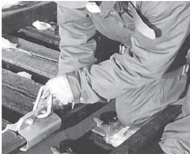
Figure 5 Profile plates are locked and secured
