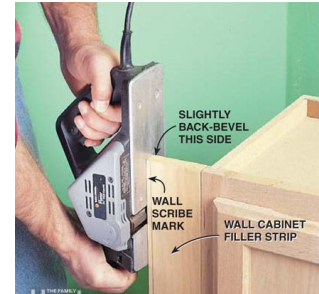
Scribing The Backs of Cabinet Side Panels and Filler Strips (5%)
