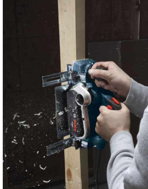
Preparing Studs & Joists for Drywall (20%)
