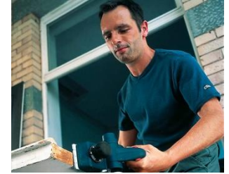
Trimming Wooden Window Frames (5%)
