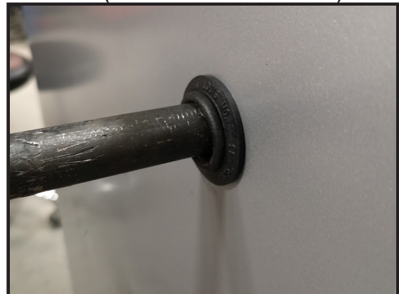
FIGURE 28 - FURNACE GAS PIPE CONNECTIONS (NOTE RUBBER GROMMET)
