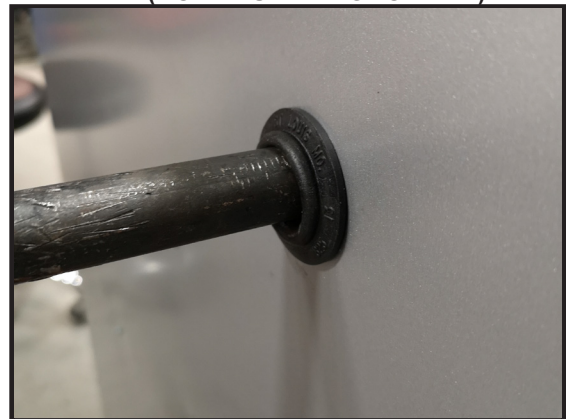
FIGURE 28 - FURNACE GAS PIPE CONNECTIONS (NOTE RUBBER GROMMET)
