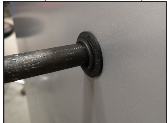
FIGURE 28 - FURNACE GAS PIPE CONNECTIONS (NOTE RUBBER GROMMET)
