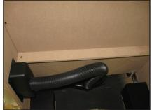
Two 2" x 1/2" MDF bottom support braces and ball return set-up. Corners of 3/8" MDF playfield are elevated.
