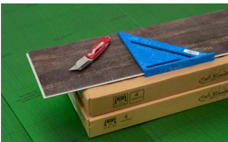
Cutting boards using Score and Snap technique
