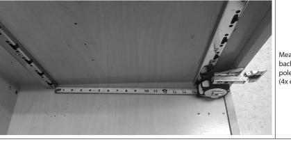
Measure 15" between front and back poles and attach back pilaster poles (A) using #8 x 1" wood screws (4x each)
