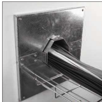
3. Push split conduit into wall.
