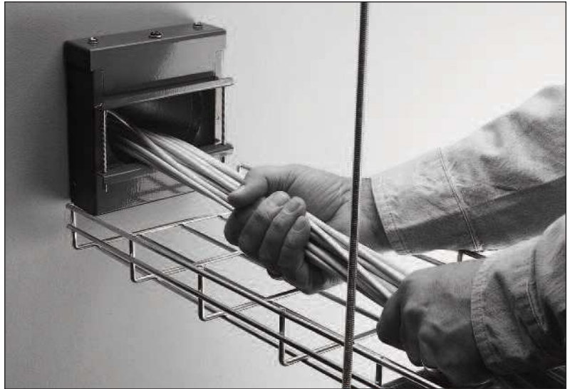
FlameStopper Thru-Wall/Floor Fittings make it easy to add cables and maintain the UL rating.
