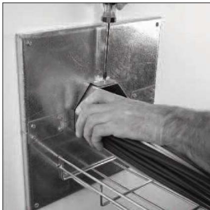
4. Screw wall plate to conduit to complete assembly.
