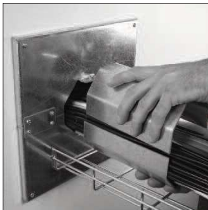
2. Attach ceramic heat protected wall plate to cover irregular hole cut. Insert split conduit around existing cables.
