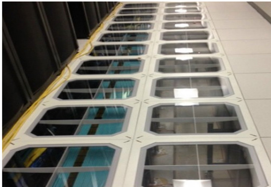
ClearView Panel Installation
